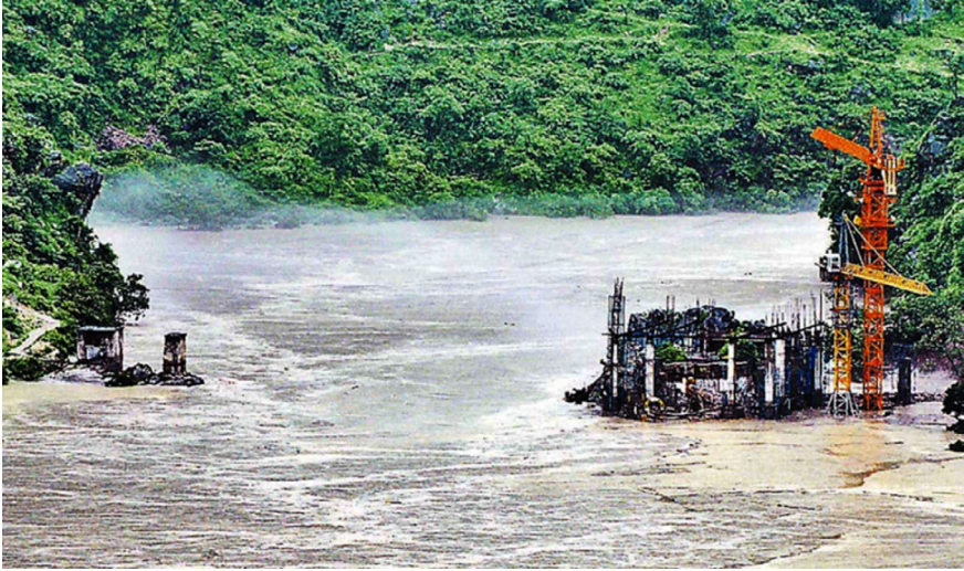
Figure 11. River, Temple and the broken Dhari Bridge in the wake of the Major Flood Event in August 2012 (Source: Amar Ujālā 2012, Aug. 5b).
