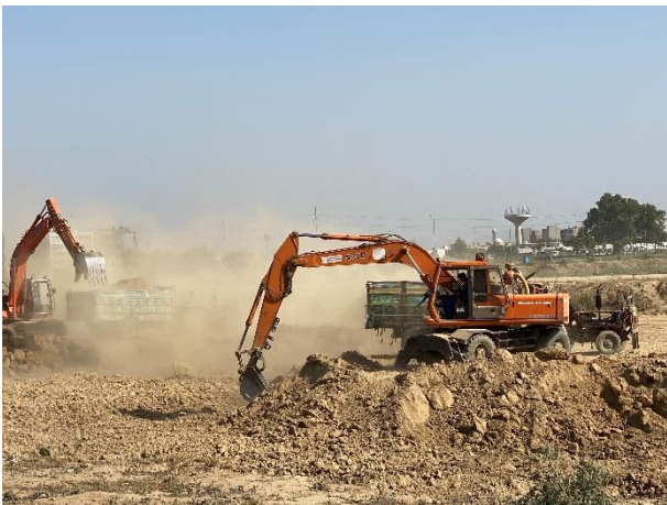
Fig. 1: Gold turning into dust. Processes of land-use change through land and soil acquisition. Five feet of village topsoil (the most fertile part) being removed for transportation to DHA (Photo: H. Javaid 2021)
