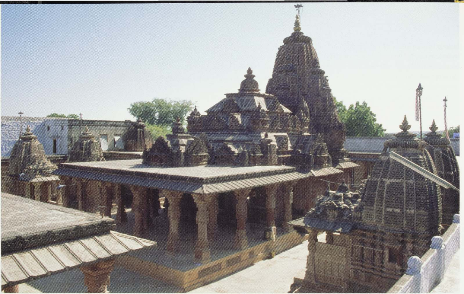
447. General view of the Mahāvīra Temple at Osian, the earliest surviving substantial temple building in the region.
