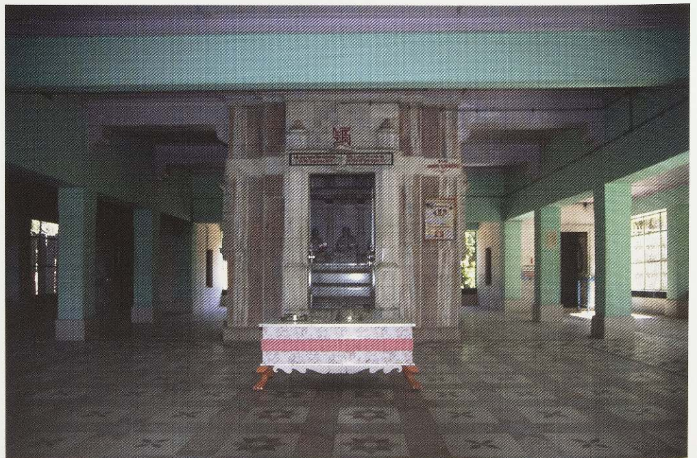
558. Variant of the hall temple type, having an enclosed shrine inserted into the open space towards the end of the hall.
