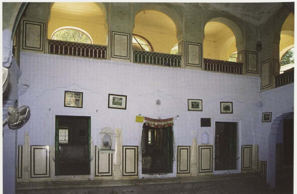
545. The Digambara Jaina Pārśvanātha Temple at the foot of Cūlagiri at Khaniyan is a roofed havelī temple. Arched openings admit light to the double-storeyed former 'courtyard' area.
