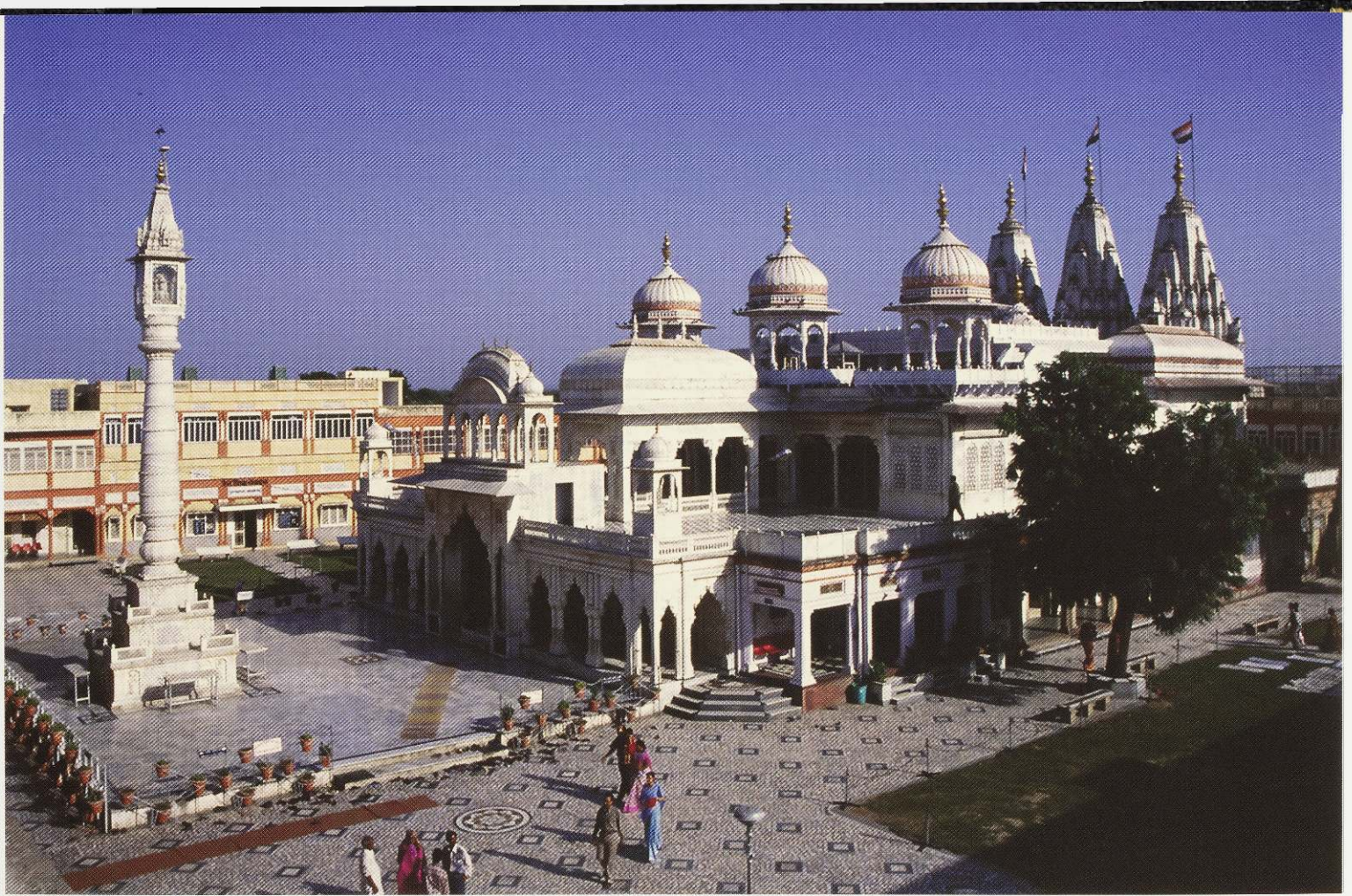
560. The Mahāvīra Temple at Mahavirji is a variant of the hall temple type. It has three aligned śikhara towers and expands over two superimposed storeys.
