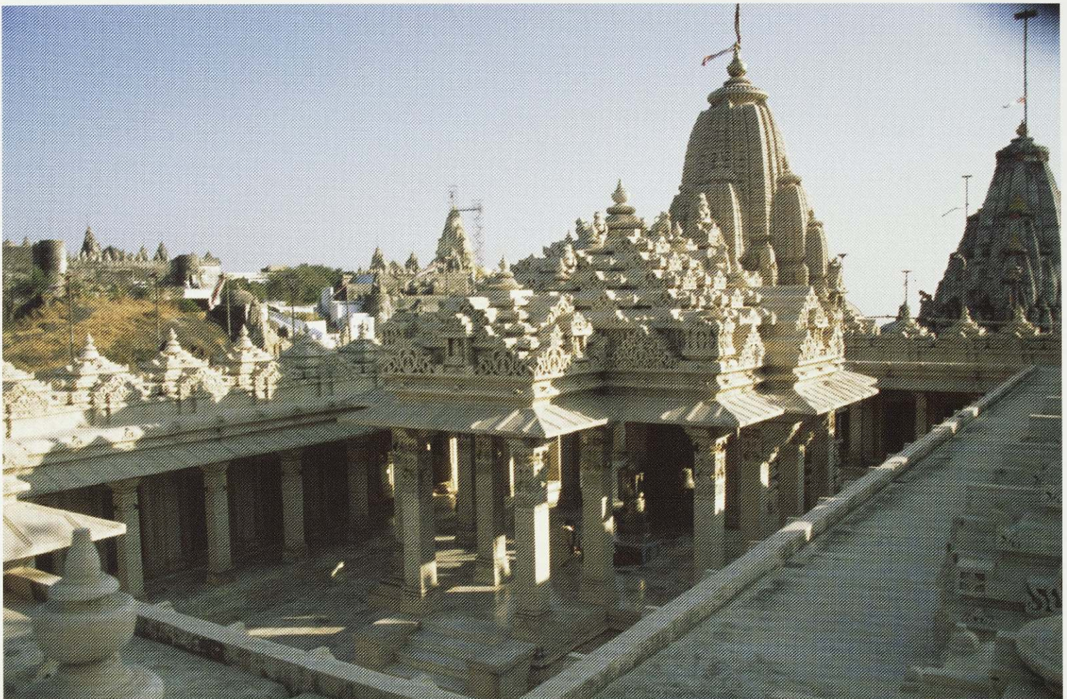
464. Temple with open hall and porch in the Nav Tunk at Palitana.
