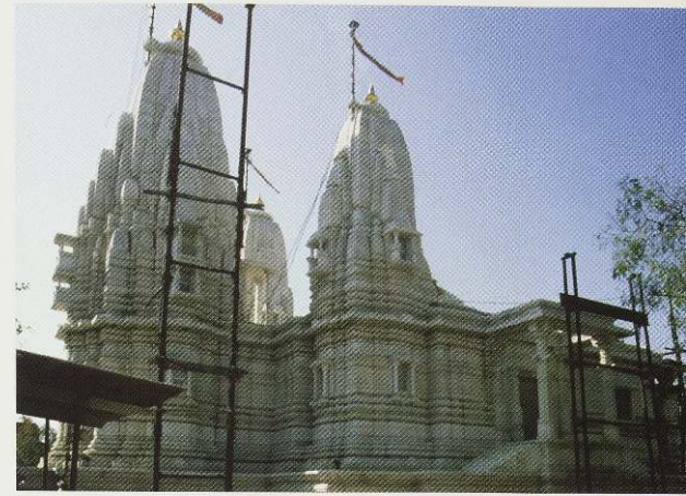
483. In the Śrī Jogivādā Śāmbājī Temple at Patan the side shrines have been positioned parallel to the central image chamber.
