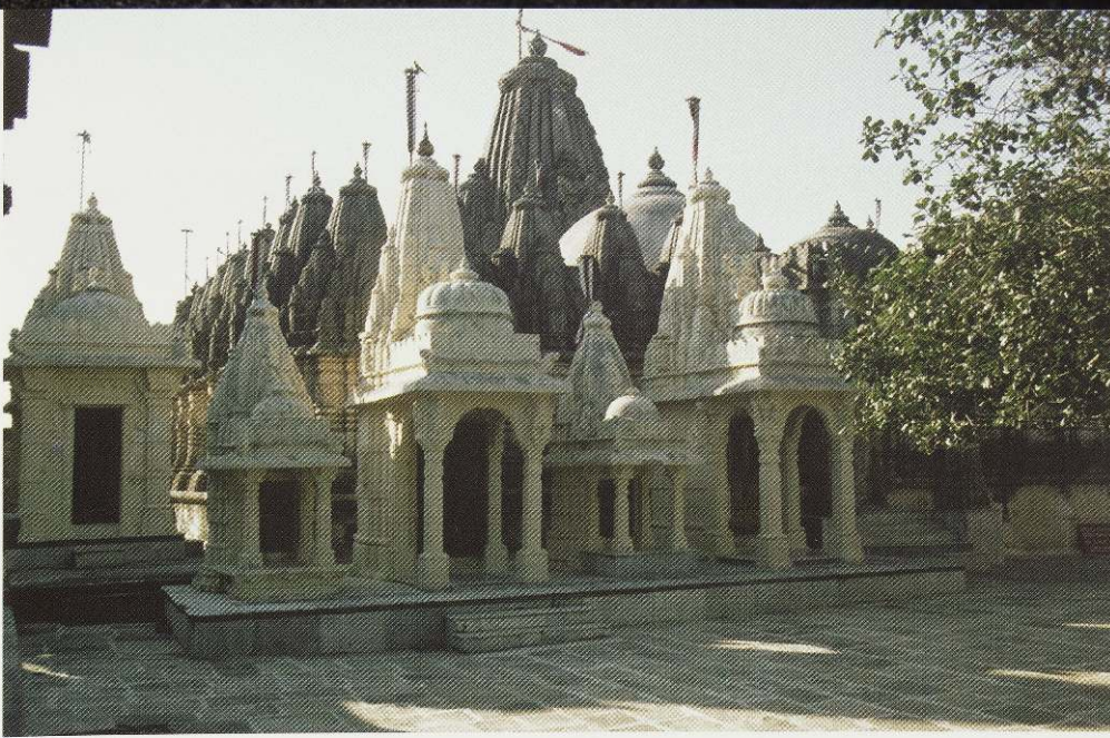
463. Subsidiary shrines preceded by open pillared porches on Mount Śatruñjaya.
