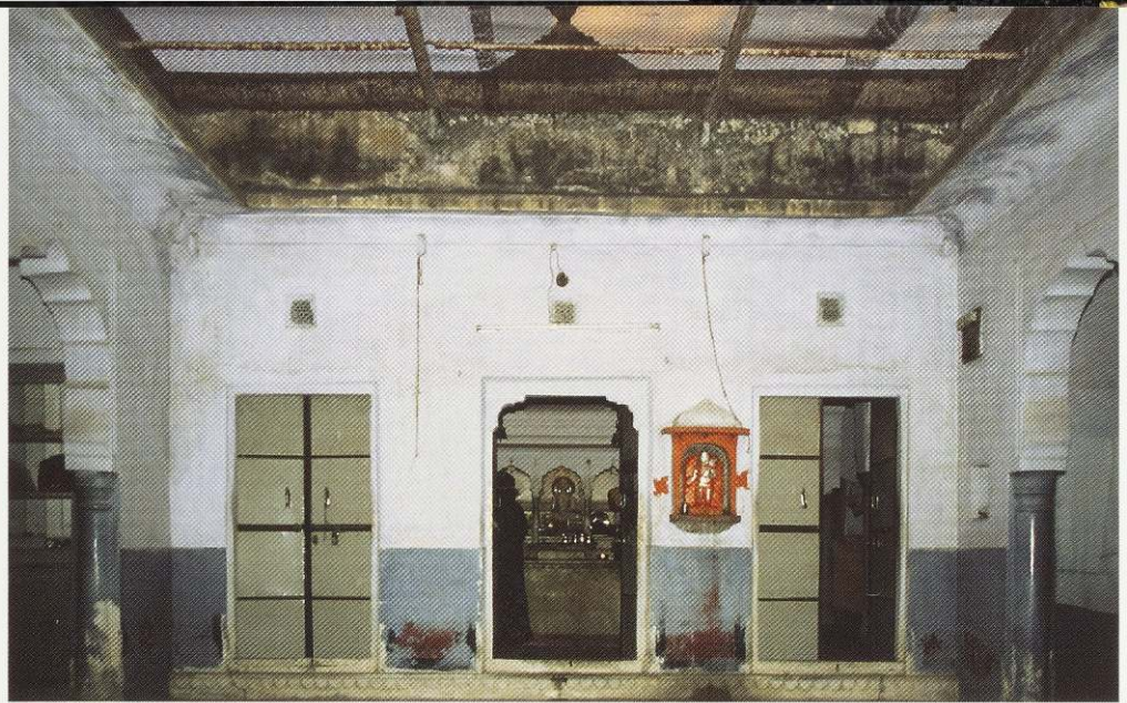
544. In the Śrī Digambra Jaina Temple at Luhadiyan, metal netting encloses the open courtyard space above.
