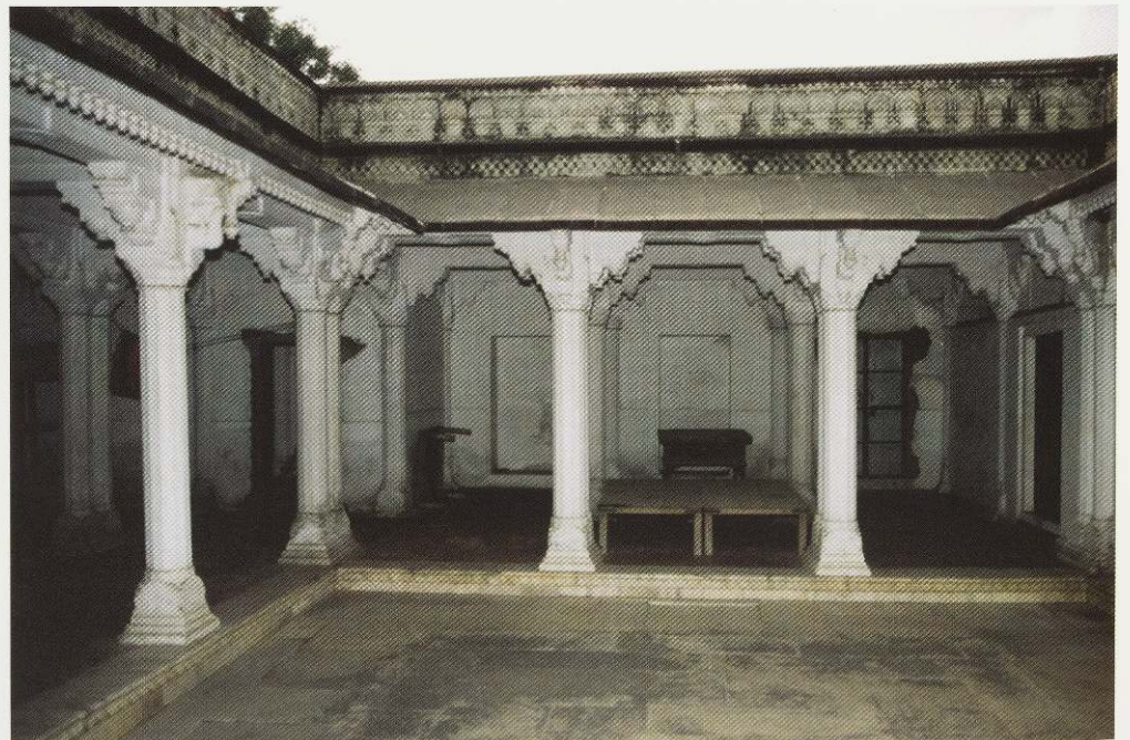
541. Double arcaded section of the cloister surrounding the open courtyard of the Digambara Jaina temple at Godikan.
