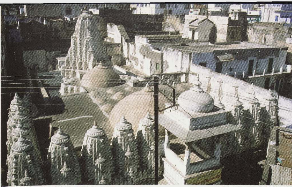
528. The Śīṭalanāthajī Mahārājikā Mandir at Udaipur combines metal meshing at the rear with a solid roof section at the front of the temple.
