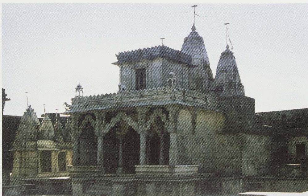
492. Temple in the Tunk of Lālcand Modī Premcand on Mount Śatruñjaya, in which an additional shrine has been raised above the temple hall.
