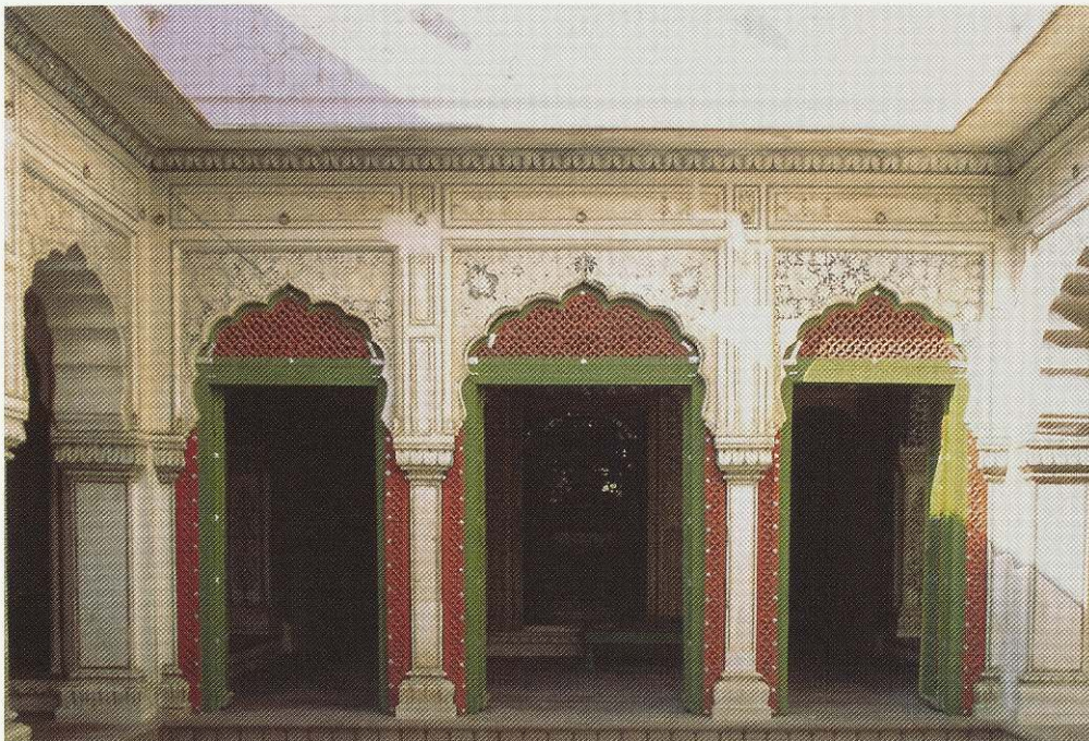
540. Arches with inserted doorways provide access to the arcade, and further doorways lead on into the shrine area of the havelī temple at Bikaner.
