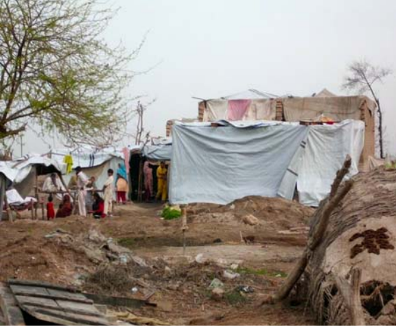
Source: photograph © Wibke Ott, February 26, 2011 Fig. 5.47: Shelter construction attached to destroyed pukka houses
