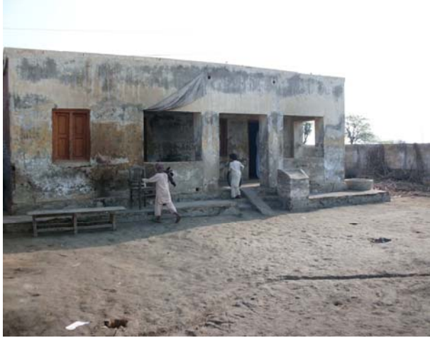
Source: photograph © Wibke Ott, February 26, 2011 Fig. 5.48: Abandoned school as shelter
