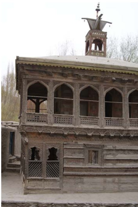
Figure 2.6 Mosque in Shigar with cribbage construction including delicate wood carvings Photo: Michel 2008
