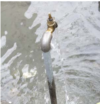
Figure 6.8 Tap without handle in Agepa
