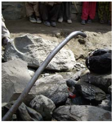
Figure 6.9 Pipe without tap in Kyahong
