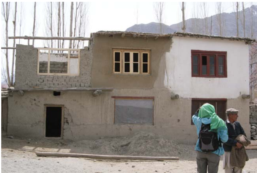
Figure 2.7 Construction stages of a building made of sun-dried adobes Photo: Michel 2008
