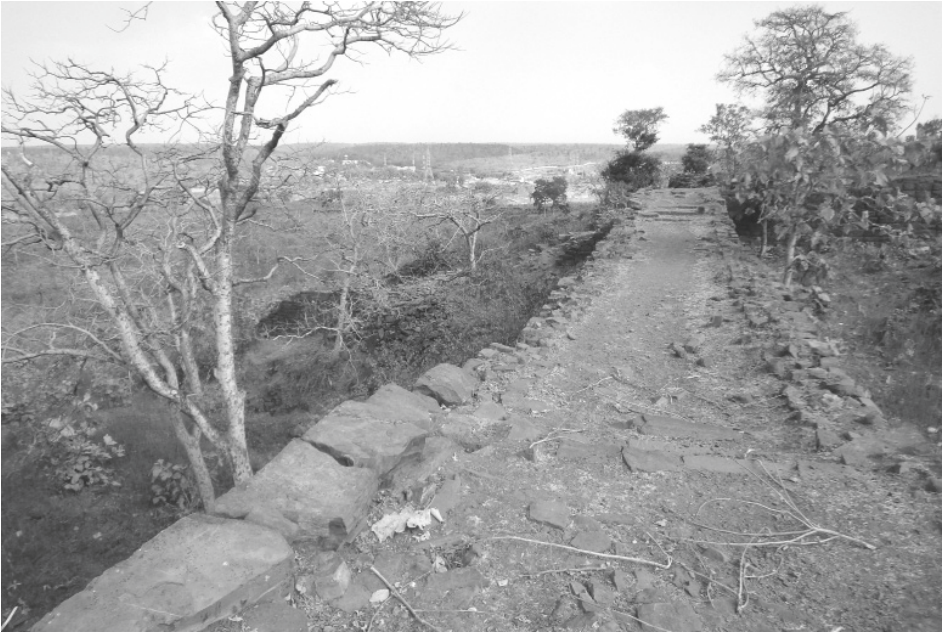
Plate 46.4: Gaurīśomanātha plateau, fortification wall near the North-east gate.
