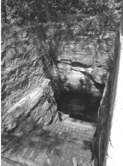
Plate 92.2: Staircase of the old well.
