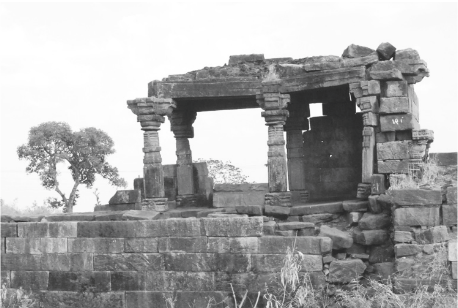
Plate 21.5: Old pillars and architraves in the upper storey of the Bhīmārjunī gate.
