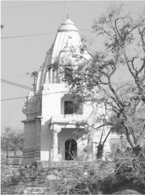
Plate 13.1: Brahmeśvara temple, general view, west side.
