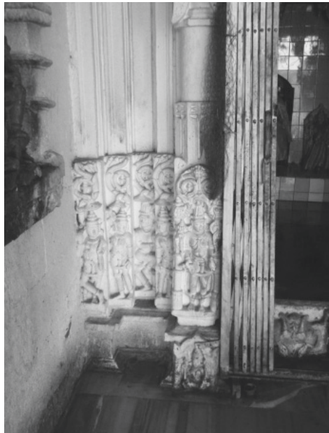
Plate 15.4: Door-frame, garbhagrha , south side.
