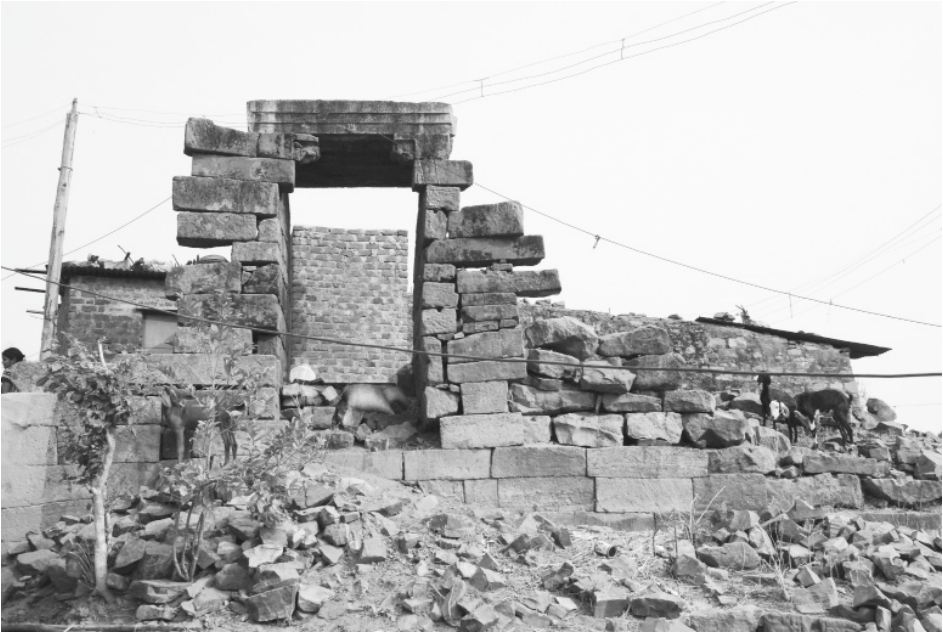
Plate 23: West gate, west side.
