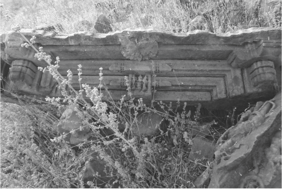
Plate 36.2: Temple C3, loose door lintel.
