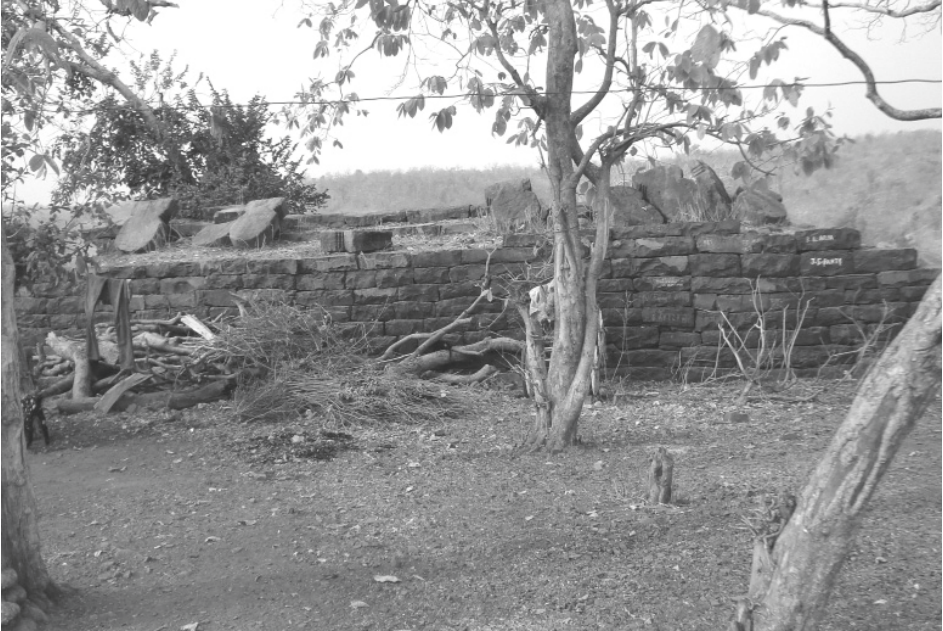
Plate 58.1: Outer fort, western section, stretch of northern outer fort wall with merlons.
