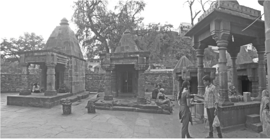
Plate 7.1: Subsidiary shrines, view from the east (nos. 3 and 4 stand to the left, behind the mandapa with Śiva's bull on the platform.)
