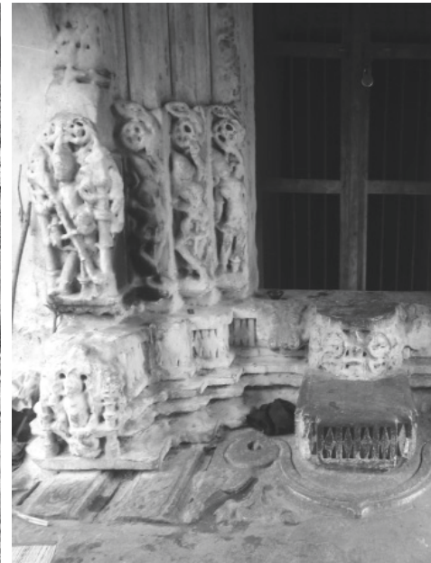
Plate 12.5: Door-frame, garbhagrha , south side.
