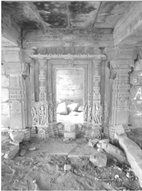
Plate 62.12: Dhavalimath, central entrance to the rear hall.
