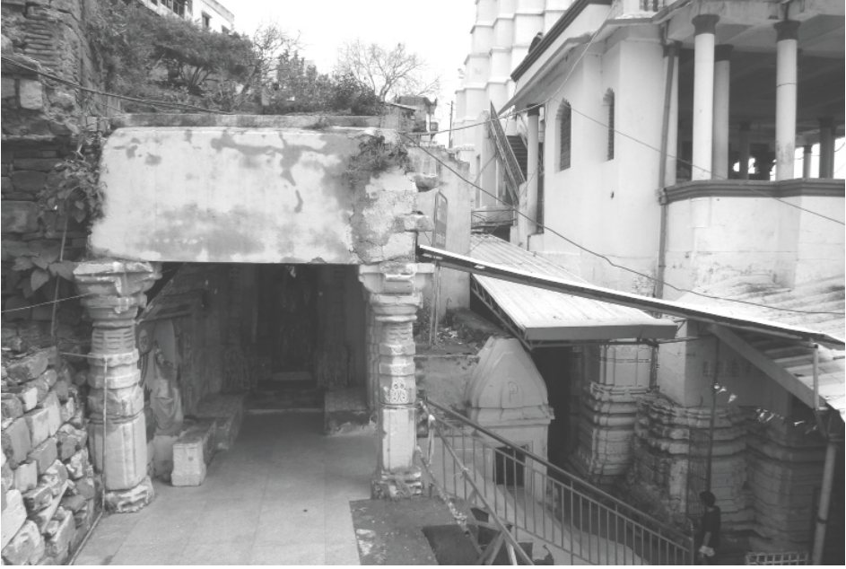
Plate 70.1: Dvārkaḍhīś, Rāṇḥoṛ temple, general view from west (with Oṃkāreśvara temple on the right side).
