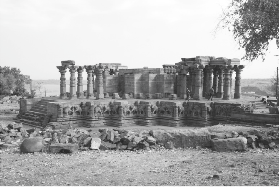
Plate 32.1: Siddhanātha temple, general view from north-west.
