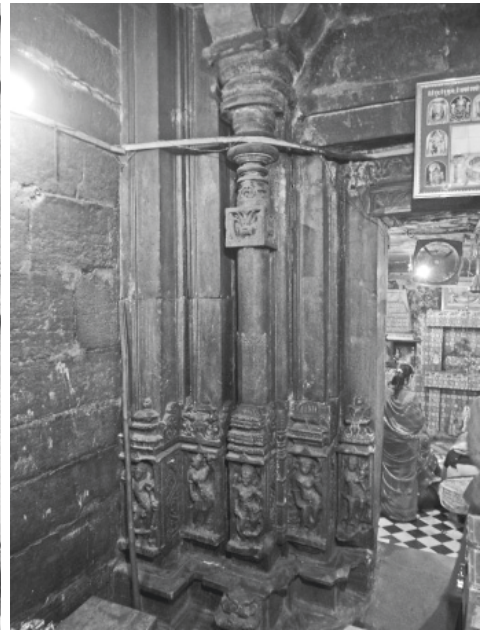
Plate 4.4: Door-frame of the garbhagrha , north (left) side.
