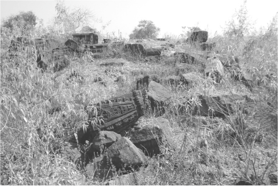
Plate 33.2: Māndhātā hill, temple B3, view from west.
