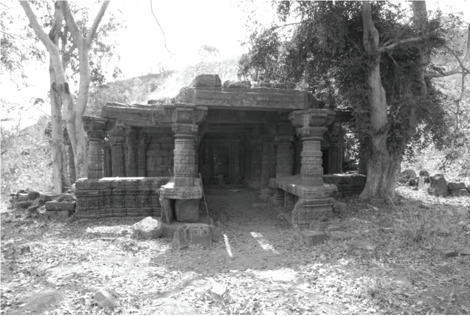
Plate 62.1: Dhavalimath, general view from north.
