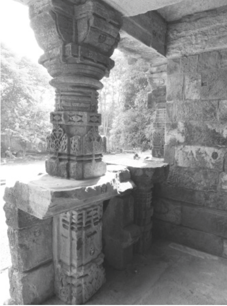
Plate 79.3: Caubis Avatār temple, 'split' pillars in balustrade of verandah.
