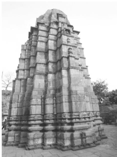
Plate 5.2: Vṛddhakāleśvara temple, north-west corner.
