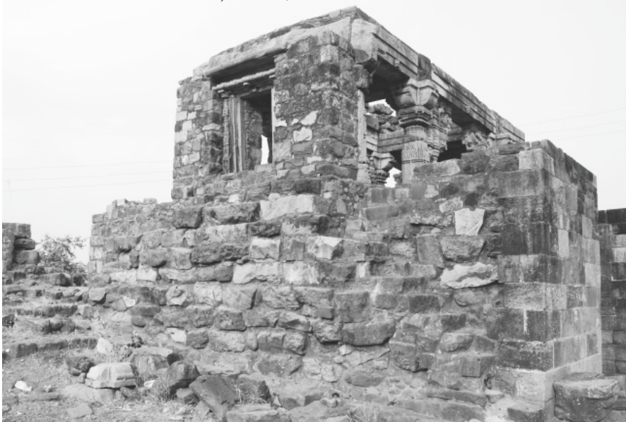
Plate 20.4: Cāndsūraj gate, west side with entrance in the upper storey.
