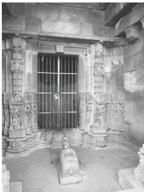
Plate 5.3: Vṛddhakāleśvara temple, entrance to the garbhagrha .
