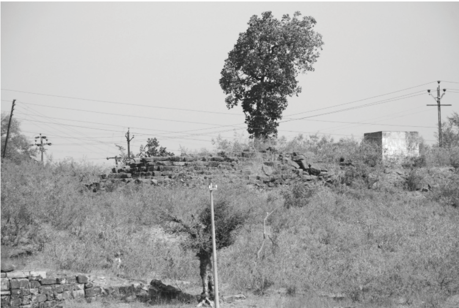
Plate 28.1: Structure A2, general view from south-west.
