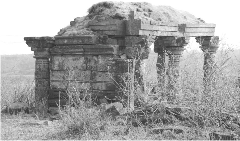
Plate 42.4: Structure E2, view from north-west.
