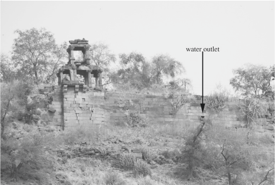
Plate 26.3: Surakṣācaukī with remains of the inner fort wall, view from south.
