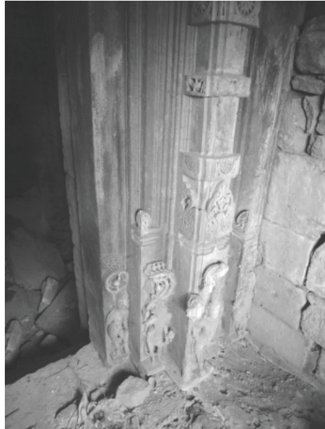
Plate 73.5: Doorframe of the garbhagrha , north side.
