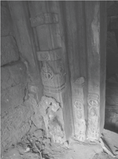
Plate 73.4: Doorframe of the garbhagrha , south side.
