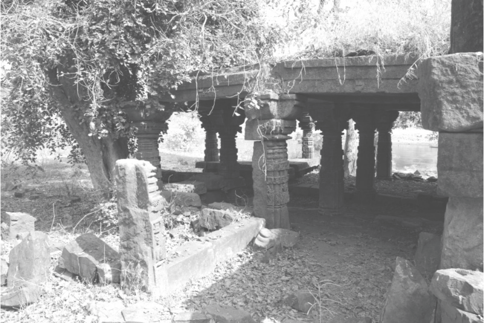
Plate 62.7: Dhavalimath, front hall, destroyed western side.
