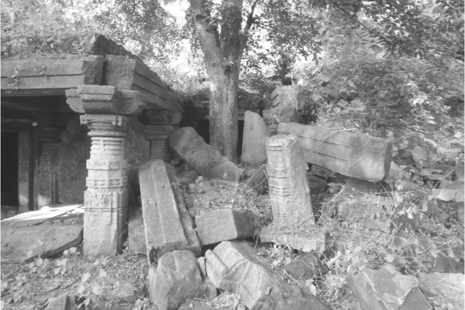
Plate 88.3: Gayāśilāmaṭh, collapsed part at the eastern side of the extant hall.
