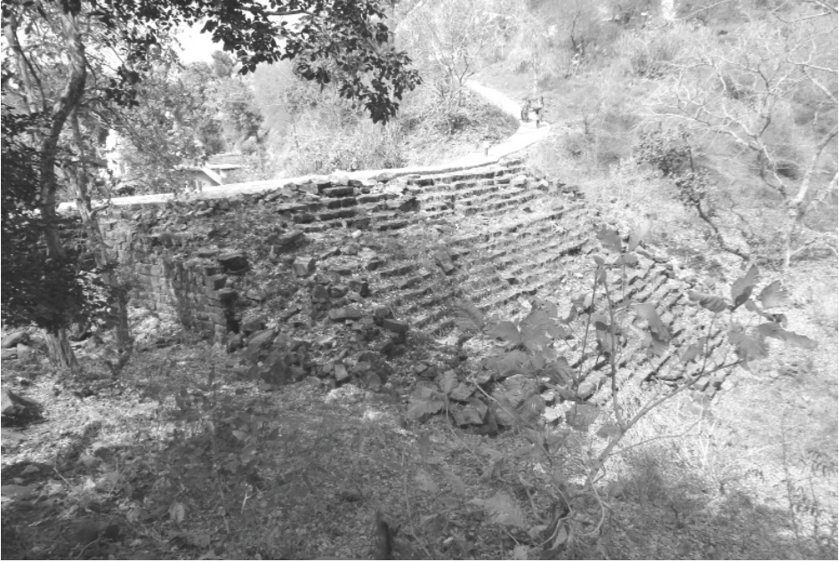
Plate 58.2: Outer fort, western section, stepped construction in the course of the outer fort wall, view from south-east.
