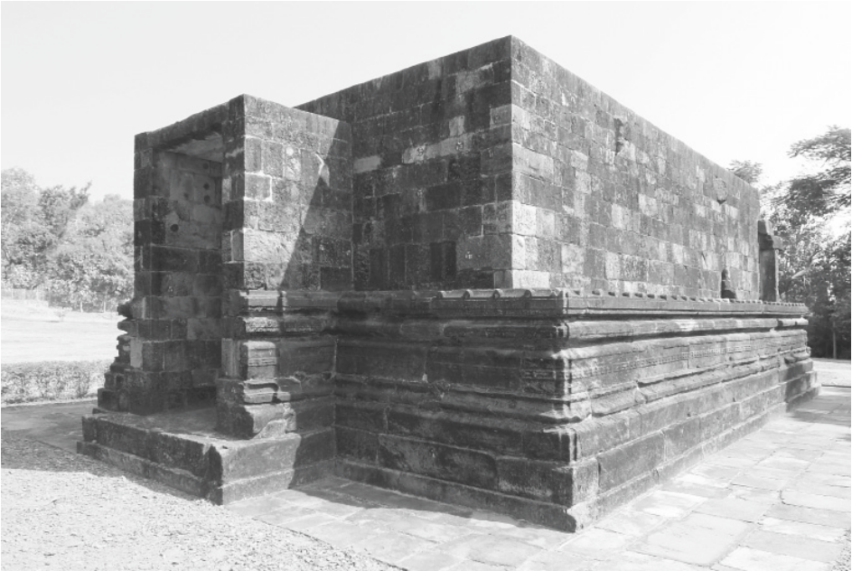
Plate 79.9: Caubīs Avatār temple, rear side, view from south-west.
