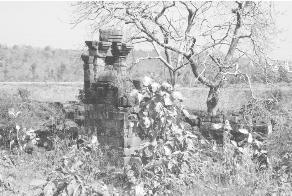
Plate 56.3: Outer fort, eastern section, East gate, view from south-east.
