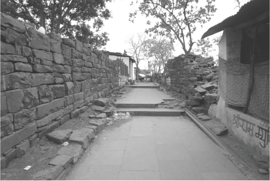
Plate 51.1: Gaurīśomanātha plateau, site No. 2, footpath with old city walls north-west of the Gaurīśomanātha temple, view from north.
