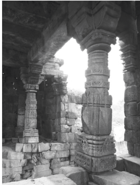
Plate 24.4: Outer north gate, western row of pillars.
