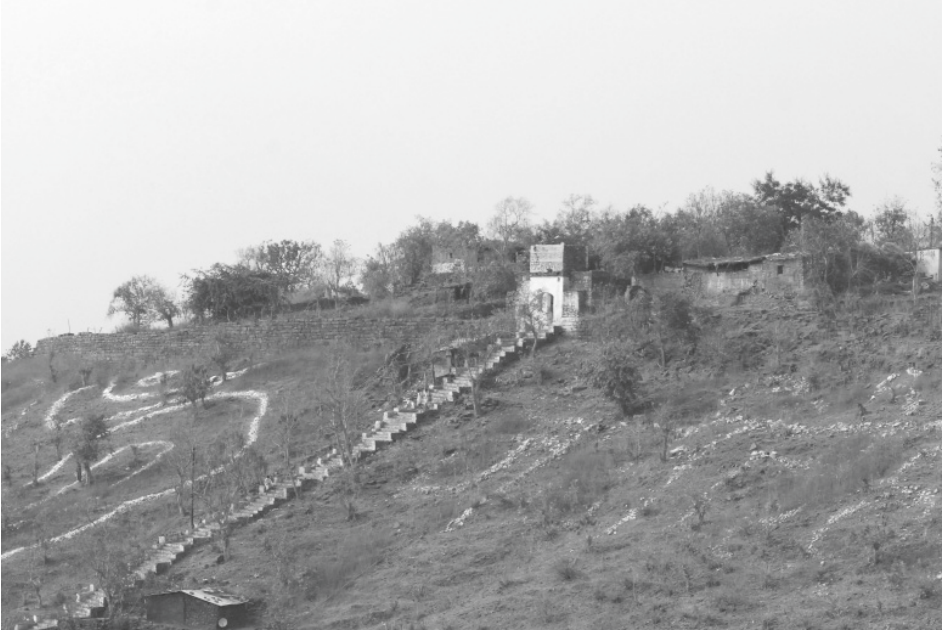
Plate 48.1: Gaurīśomanātha plateau, South gate and staircase, general view from south-east.
