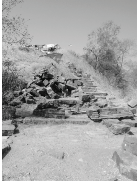
Plate 19.2: Platform B3, view from east.
