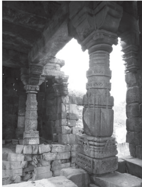
Plate 24.4: Outer north gate, western row of pillars.
