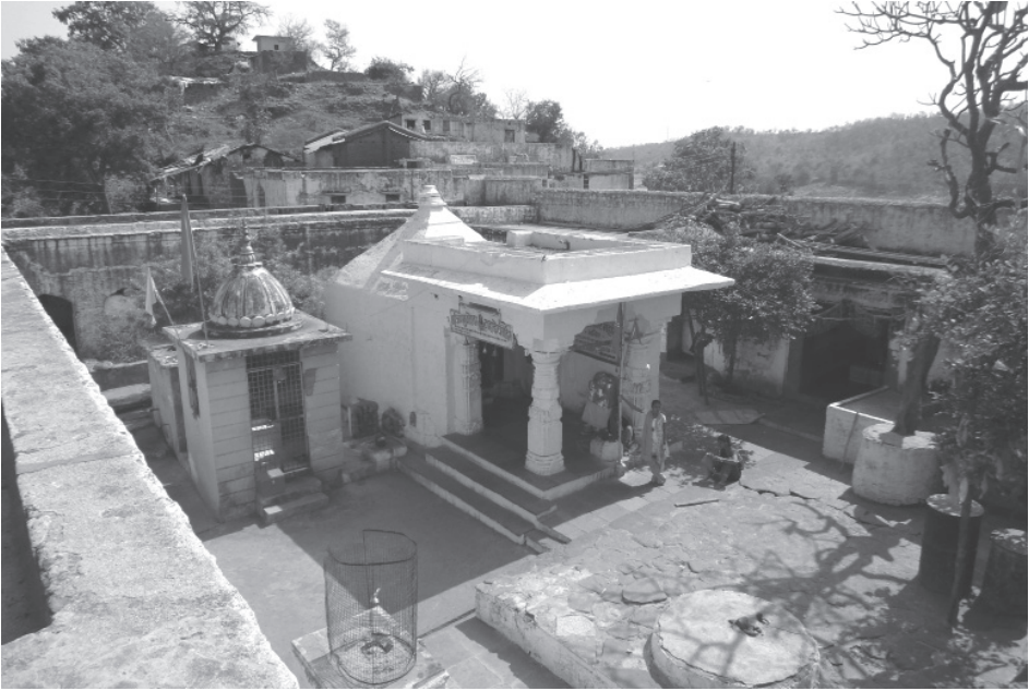
Plate 60.1: Āṇamukteśvara temple, view from north-west.
