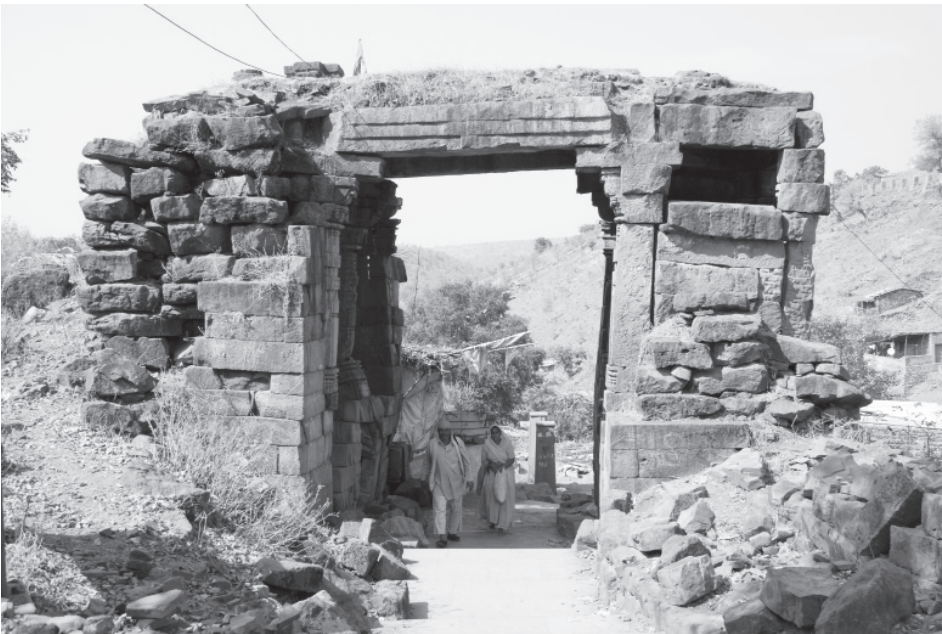
Plate 24.1: Outer north gate, view from south-east.
