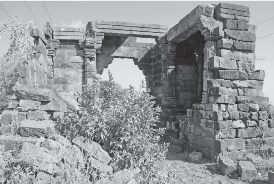
Plate 25.2: Inner or Huṇḍī-kuṇḍī gate, west side.
