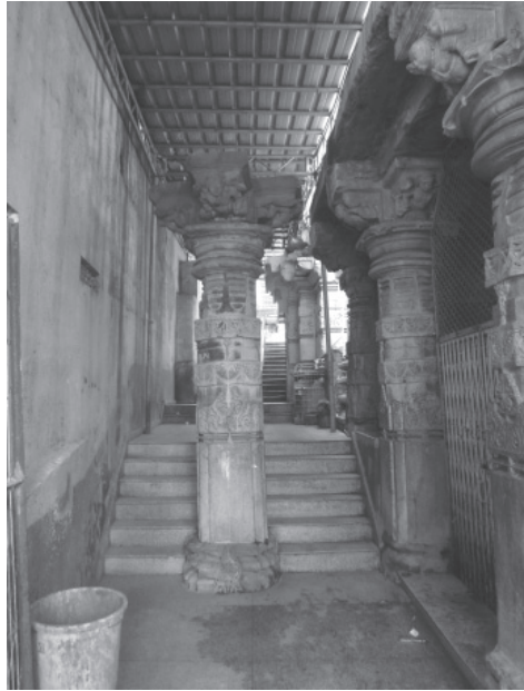
Plate 69.9: Omkāreśvara temple, northern mukhamaṇḍapa , view from west.
