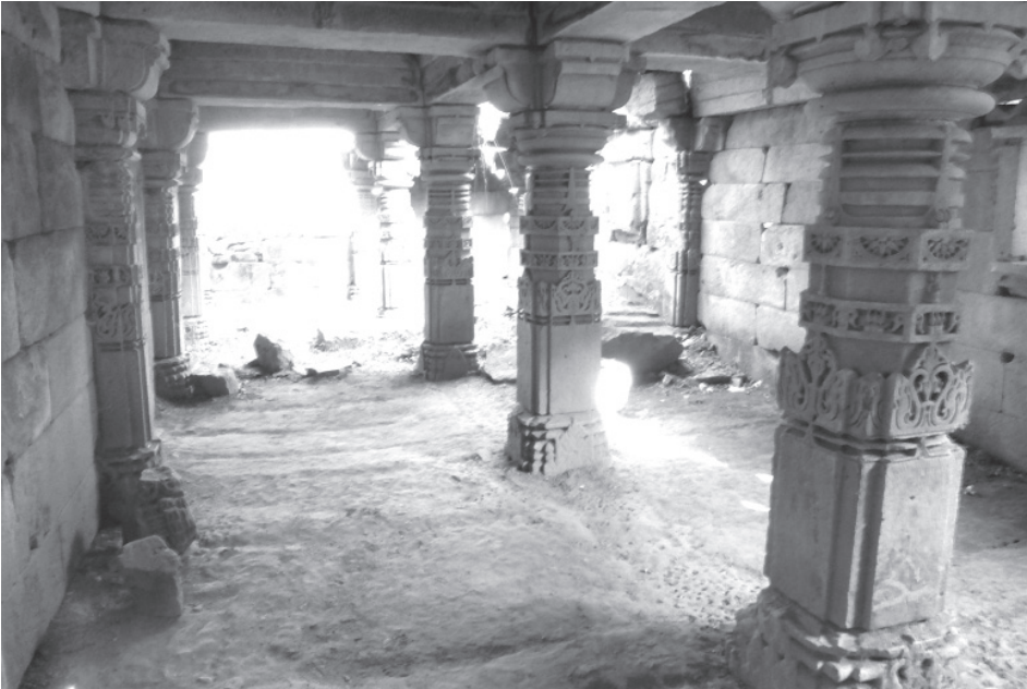
Plate 62.26: Dhavalimath, rear hall, east side (eastern wall partly collapsed).
