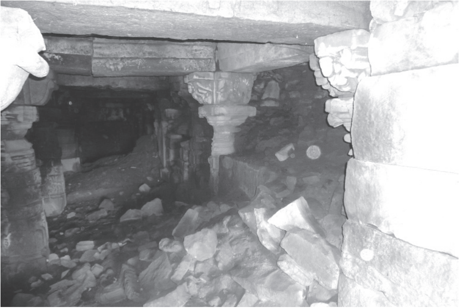
Plate 71.11: 'Old mahal' look into the large pillared hall with debris.
