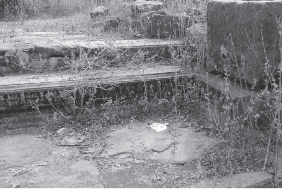
Plate 52.6: Gaurīśomanātha plateau, site No. 3, temple platform, grāsapaṭṭī base moulding.
