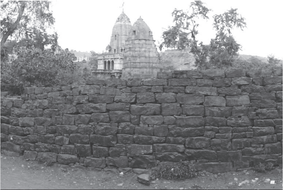
Plate 3.2: Fortification wall to the west of the Amareśvara temple complex.
