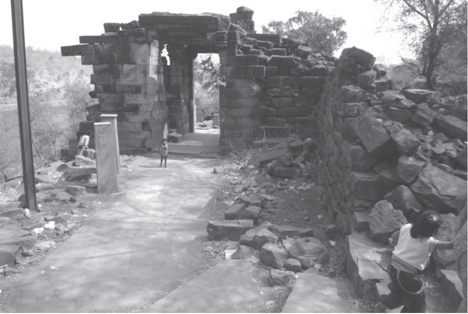
Plate 58.4: Outer fort, western section, Dharmrāj gate, view from west.
