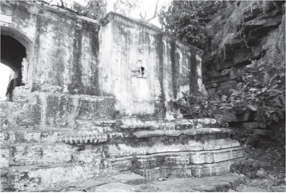
Plate 12.3: Kapileśvara temple, mūlaprāsāda , north side.
