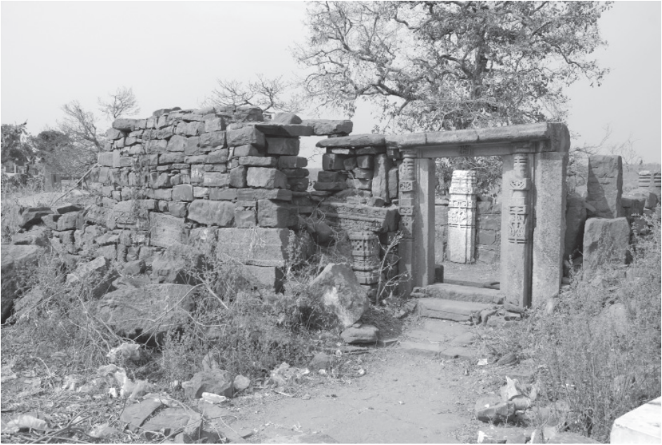
Plate 52.2: Gaurīśomanātha plateau, site No. 3, 'structure', general view from south-east.
