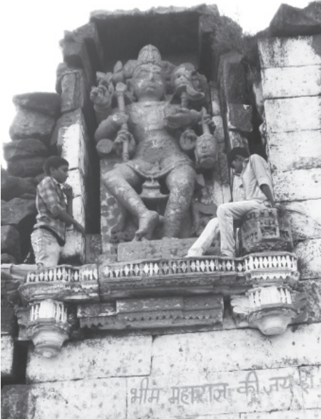
Plate 21.7: Bhīmārjunī gate, front wall, south niche.
