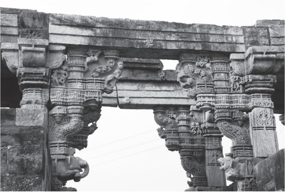
Plate 20.5: Cāndsūraj gate, pratolī toraṇas , view from south.
