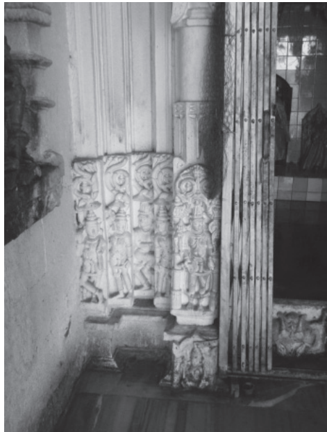
Plate 15.4: Door-frame, garbhagrha , south side.
