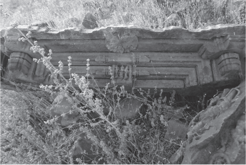
Plate 36.2: Temple C3, loose door lintel.
