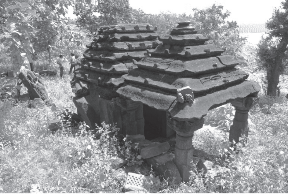
Plate 90.2: Phamsanā shrine, general view from north-west.
