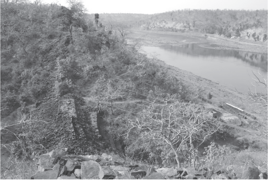
Plate 57: Outer fort, central section, detail of northern outer fortification wall traversing a valley.
