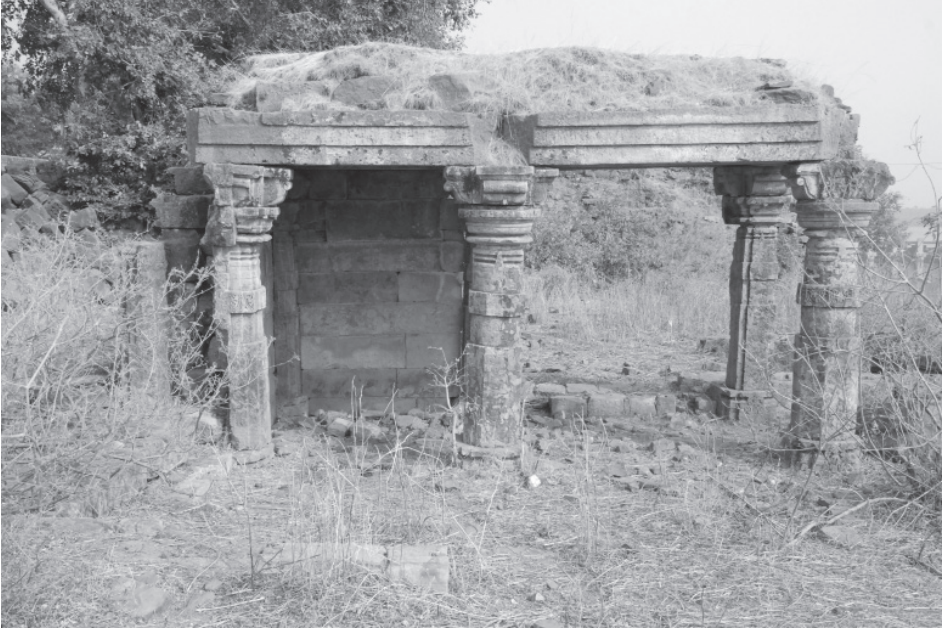
Plate 42.2: Structure E2, general view, west side.
