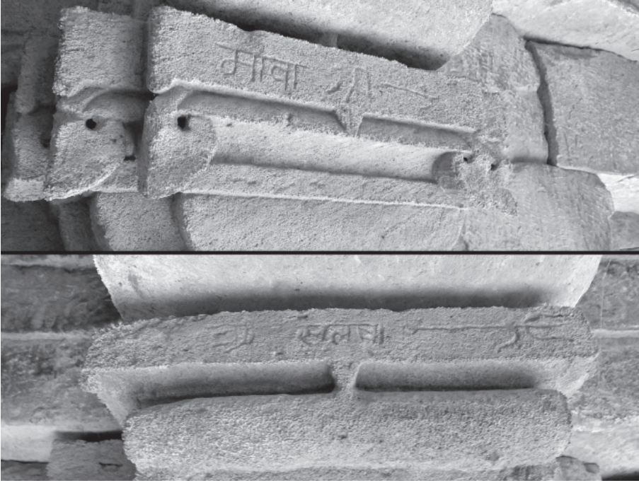
Plate 62.27: Dhavalīmaṭh, rear hall, inscriptions on a pillar and a pilaster.
