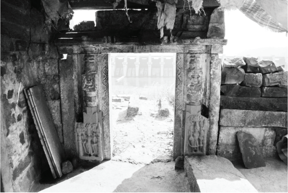
Plate 18.2: Structure B2, old door-frame in the eastern wall.
