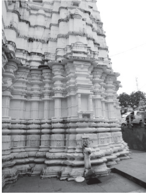
Plate 15.2: Viṣṇu temple, mūlaprāsāda , north side.
