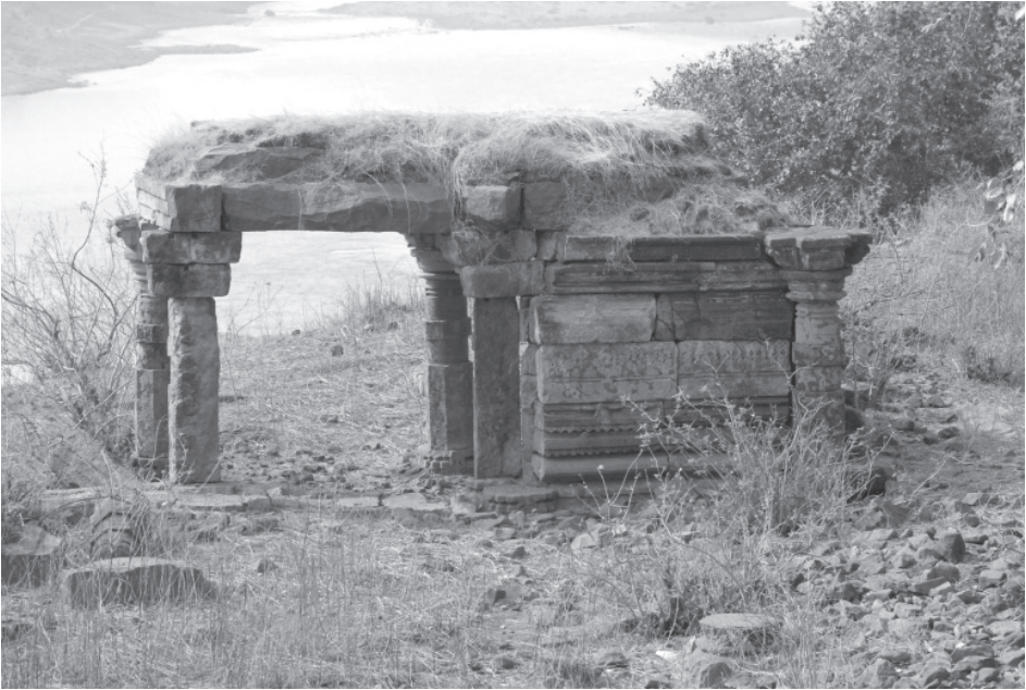
Plate 42.1: Structure E2, general view, east side.
