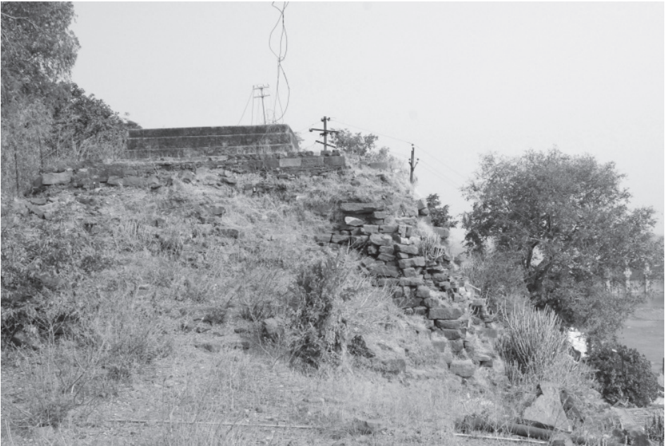
Plate 40.3: Remains of fort wall and rectangular platform at the south-eastern edge of area E.
