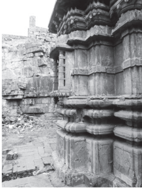
Plate 10.4: Indreśvara temple, maṇḍovara , north side.
