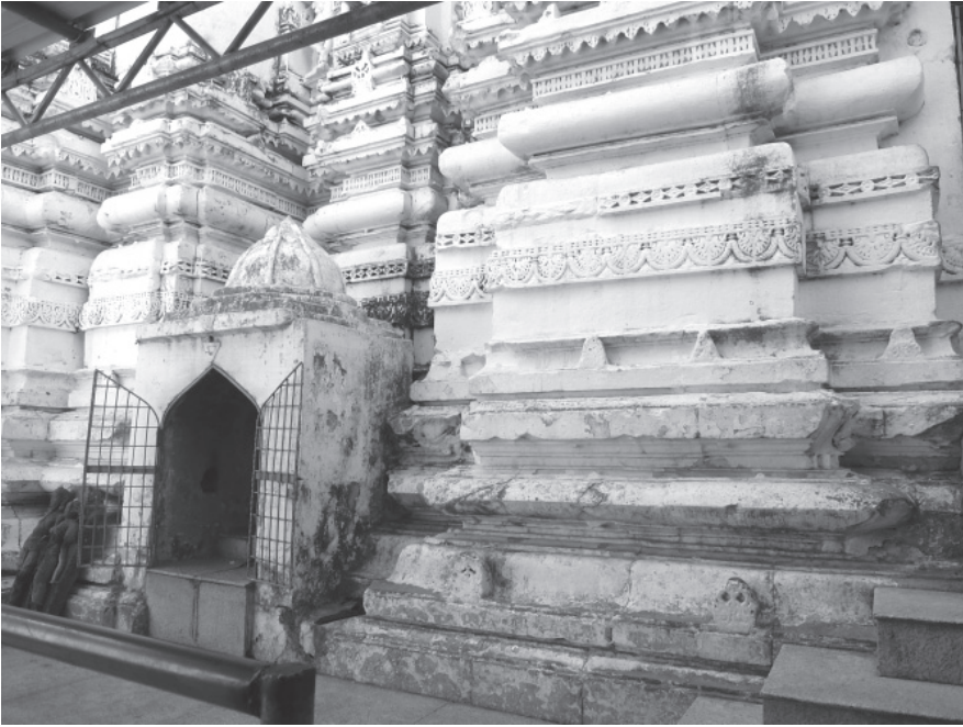
Plate 69.4: Omkāreśvara temple, base and wall of the mūlaprāsāda , north side (view from below).
