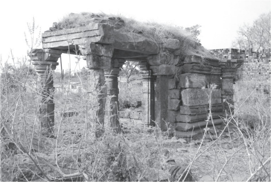
Plate 42.3: Structure E2, south-east corner.
