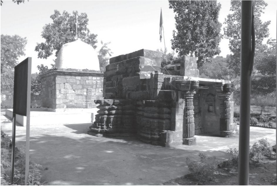
Plate 82.1: Śiva and Paśupatinātha temples at their relocation site, view from north-west.
