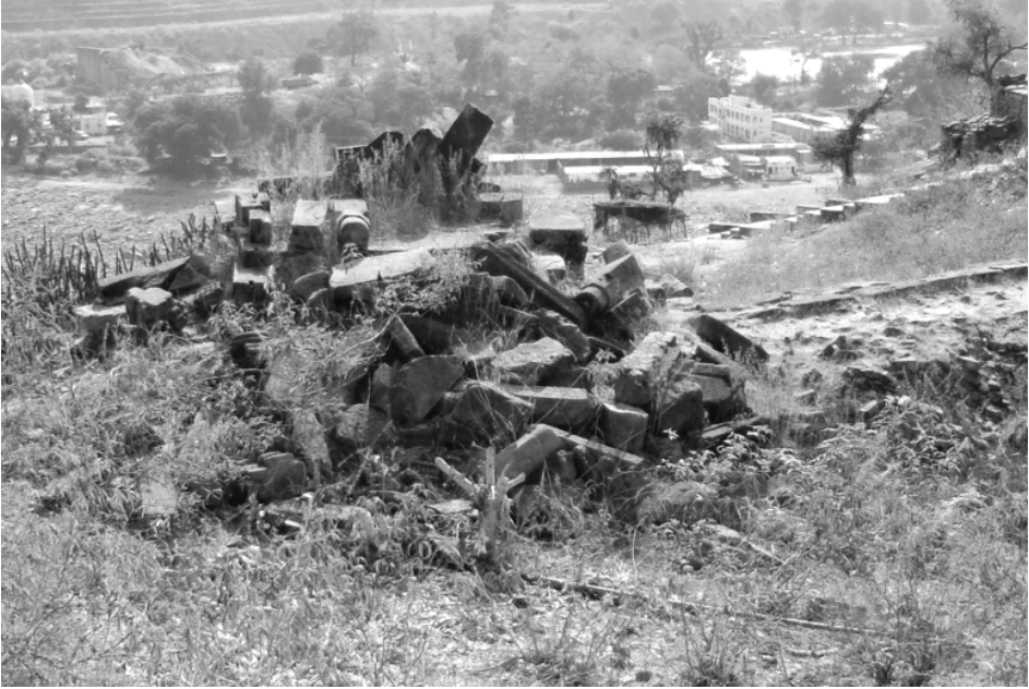
Plate 26.2: Platform near Bhīmārjunī gate with remains of a collapsed building, view from north-west.
