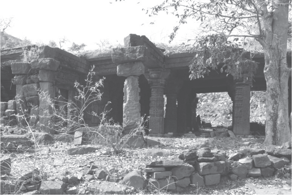
Plate 62.6: Dhavalimath, front hall, destroyed eastern side.
