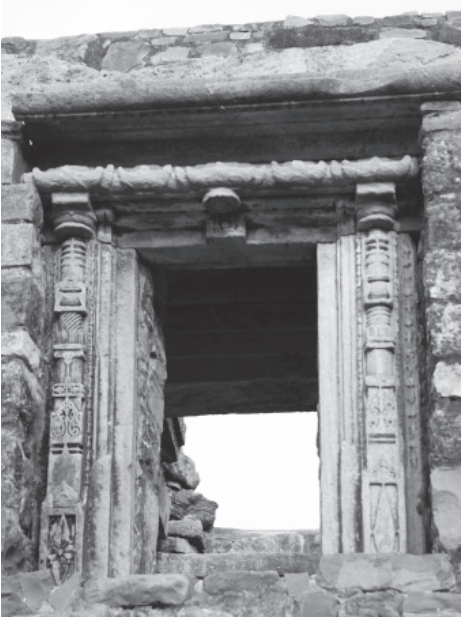
Plate 20.7: Cāndsūraj gate, door-frame in the upper storey, west side.
