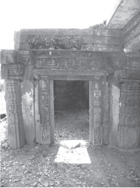
Plate 62.10: Dhavalimath, western entrance to the rear hall.
