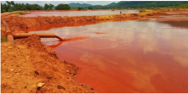
Fig. 3: Tailings dam used for slurry deposits in Kadampal, Chhattisgarh (photo: M. Chaturvedi 2017)
