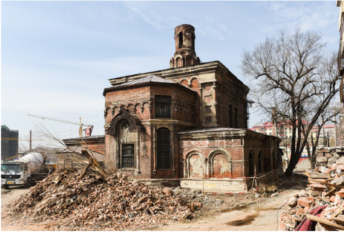
Figure 14-15: Restoration starting with clearance of the surrounding area – April 13, 2017 20
