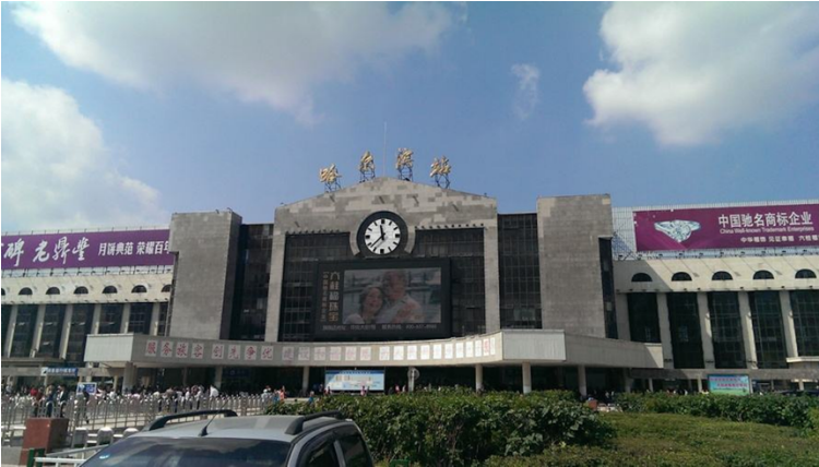
Figure 14-32: The Harbin Railway Station in 1988 photo taken by Li Suian
