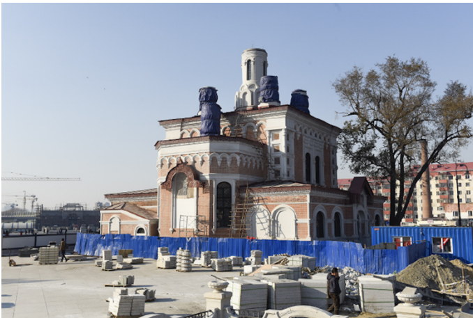
Figure 14-16: Restoration of the exterior finished first without the domes – October 25, 2017 21
