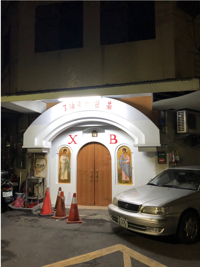
Figure 13-1: Church building in November 2018 Photo taken by Min-Chin Kay CHIANG
