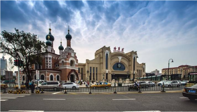
Figure 14-20: The restored Holy Iveron Icon Orthodox Church and the newly built North Square of Harbin Railway Station 25
