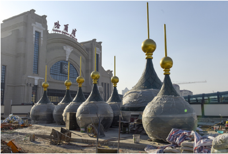
Figure 14-17: Seven wrought onion shaped domes waiting to be mounted 22
