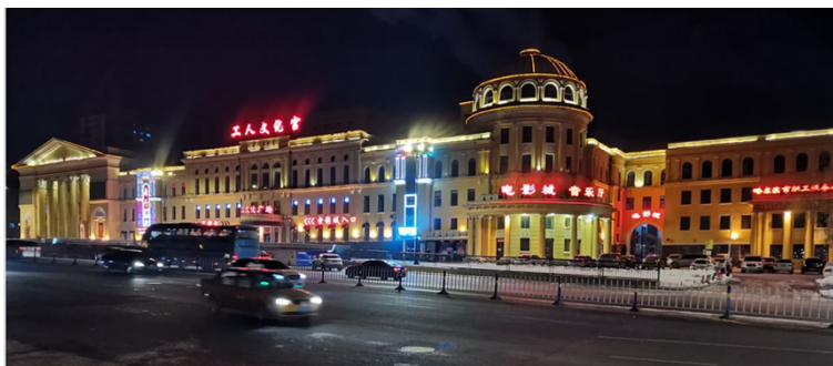
Figure 14-3: The Harbin Workers Cultural Palace Photo taken by LI Suian
