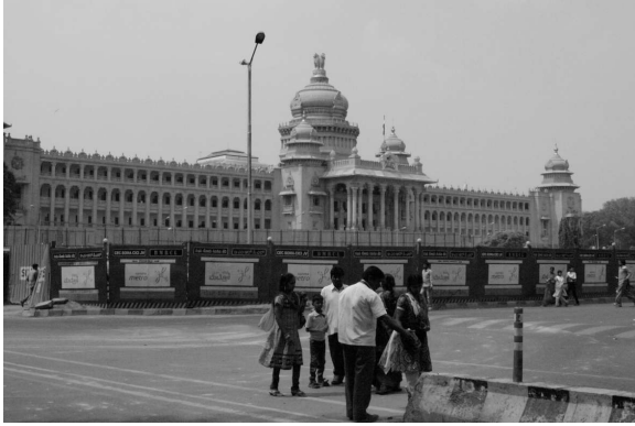
The Vidhana Soudha, seat of Karnataka's Legislative Assembly, Bengaluru: the largest legislative building in India
