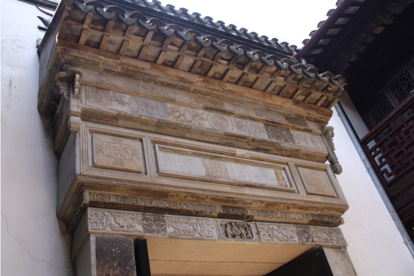
Figure 4-21. Engraved Archway of Jiayin Hall.
