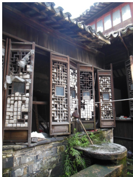
Figure 4-8. Windows with Transparent Oyster Shells.
