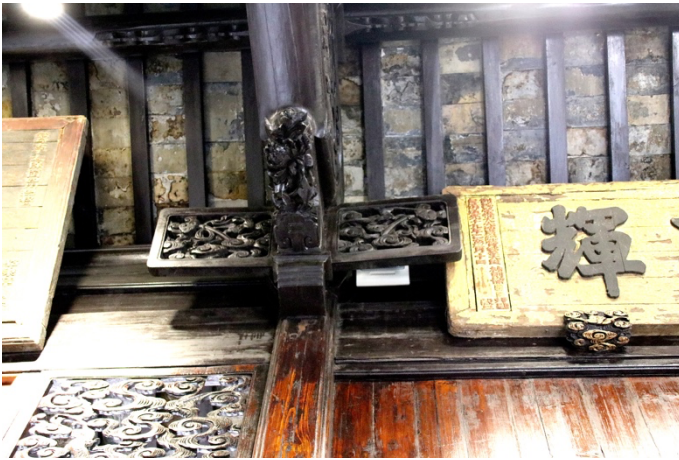
Figure 3-12. Engraved Zhaomu in Former Residence of Pan Shi'en (from below).
