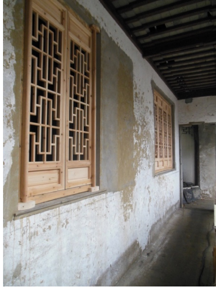
Figure 4-33. Substitution of Wooden Windows.
