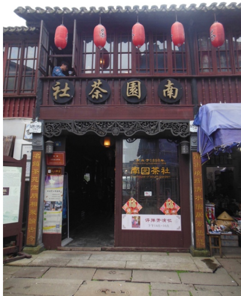
Figure 4-28. Restored Nanyuan Teahouse.
