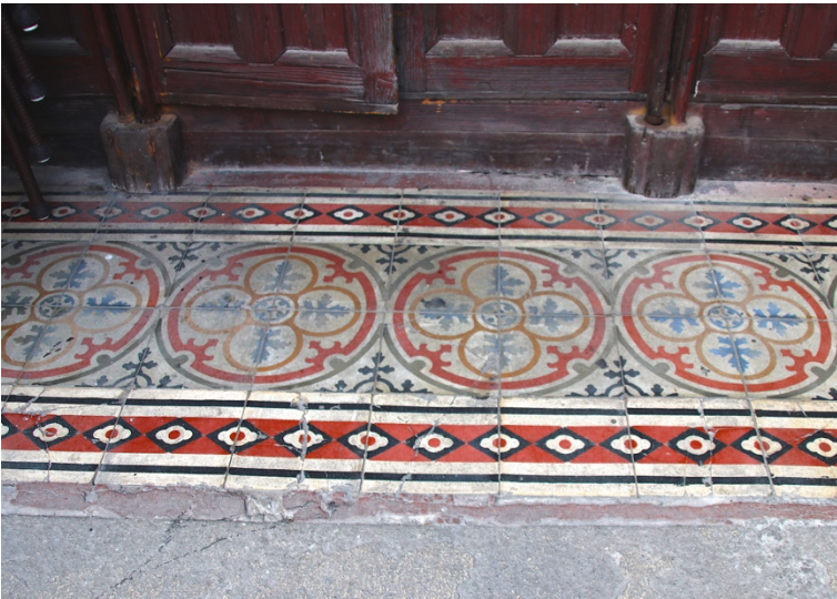
Figure 3-14. Colored Floor Tiles of Republican Period Building.
