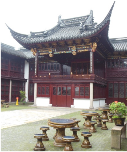
Figure 3-5. Quan-Jin Guild Hall Opera Building in Shanxi Style.
