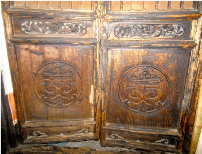
Figure 4-10. Wooden Carvings on Door Panels.
