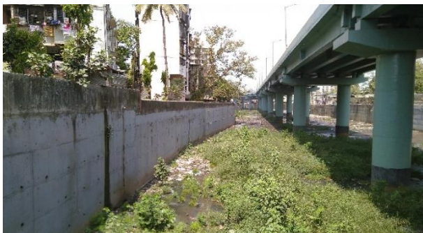
Fig. 2: Flood retention wall in Mumbai's northwestern suburb Dahisar (Photo: T. Zimmermann 2019)
