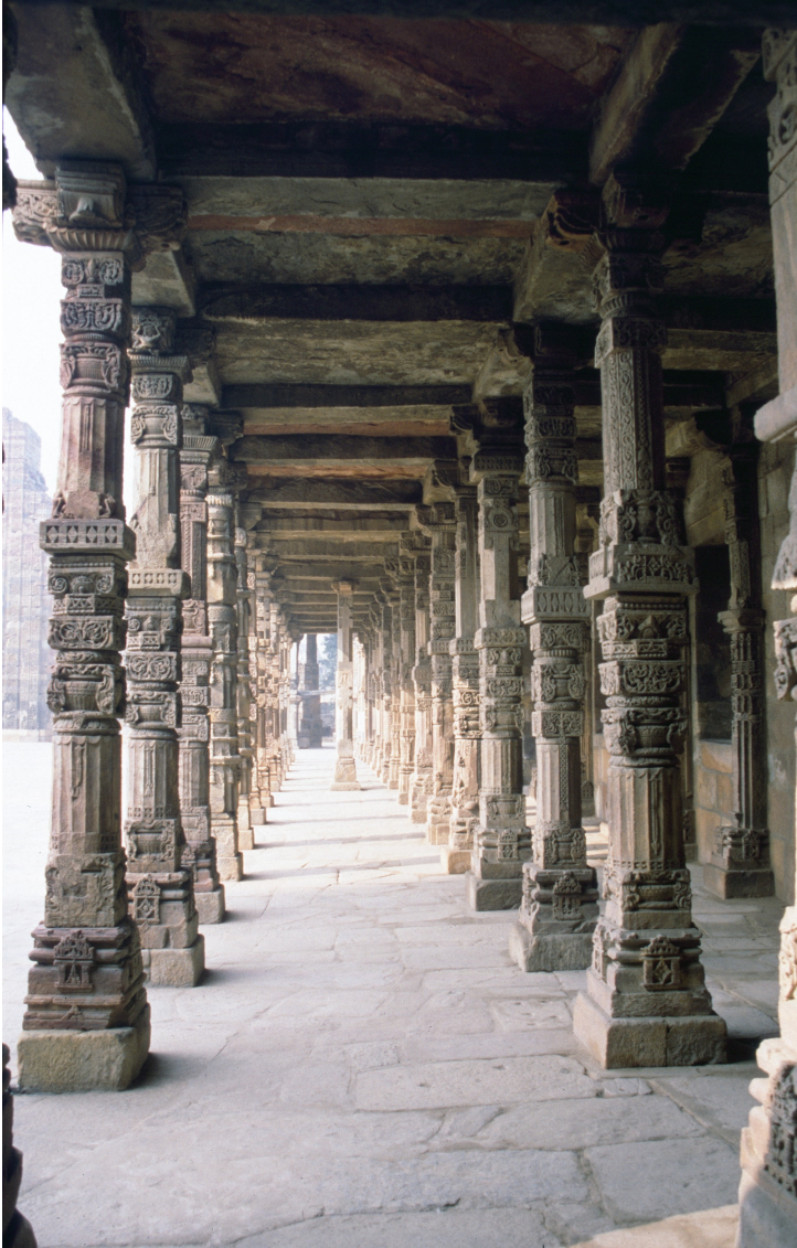
Plate 2: Two pillared-up re-used Hindu and Jaina pillars have been used to form the prayer hall and the arcading of the Quwwatu'l Islām Mosque in Delhi.
