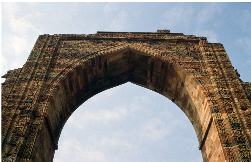
Plate 8: Although the arches look arcuate, they have been created by superimposing horizontal stone courses and cutting off the cantilever ends.
