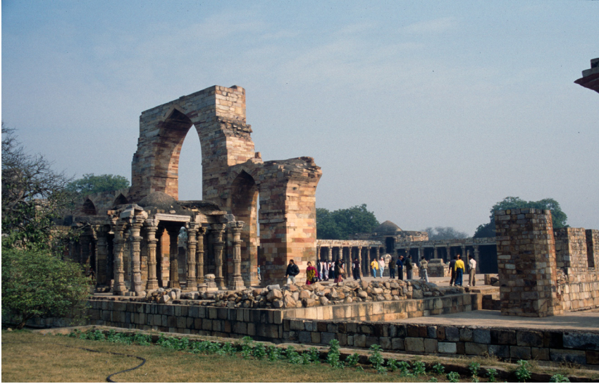
Plate 7: View onto the back of the earlier columned prayer hall with flat ceilings raised out of temple debris and the later much taller screen of arches.
