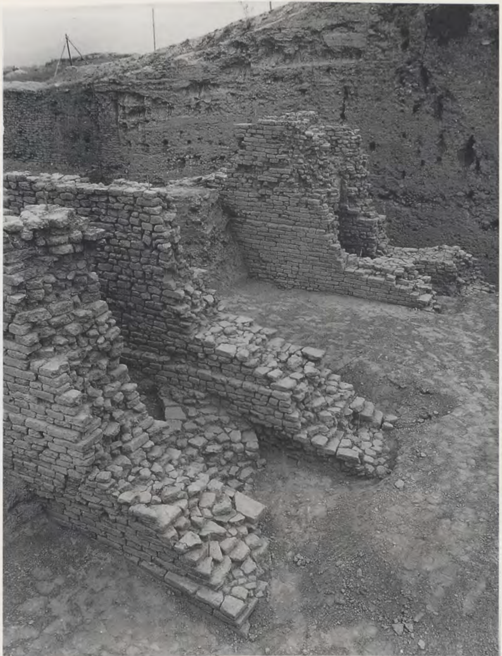
72 Remains of fortress porch with earlier tower under left wing
