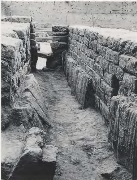
43 Level 26: Drain between Blocks E and F
