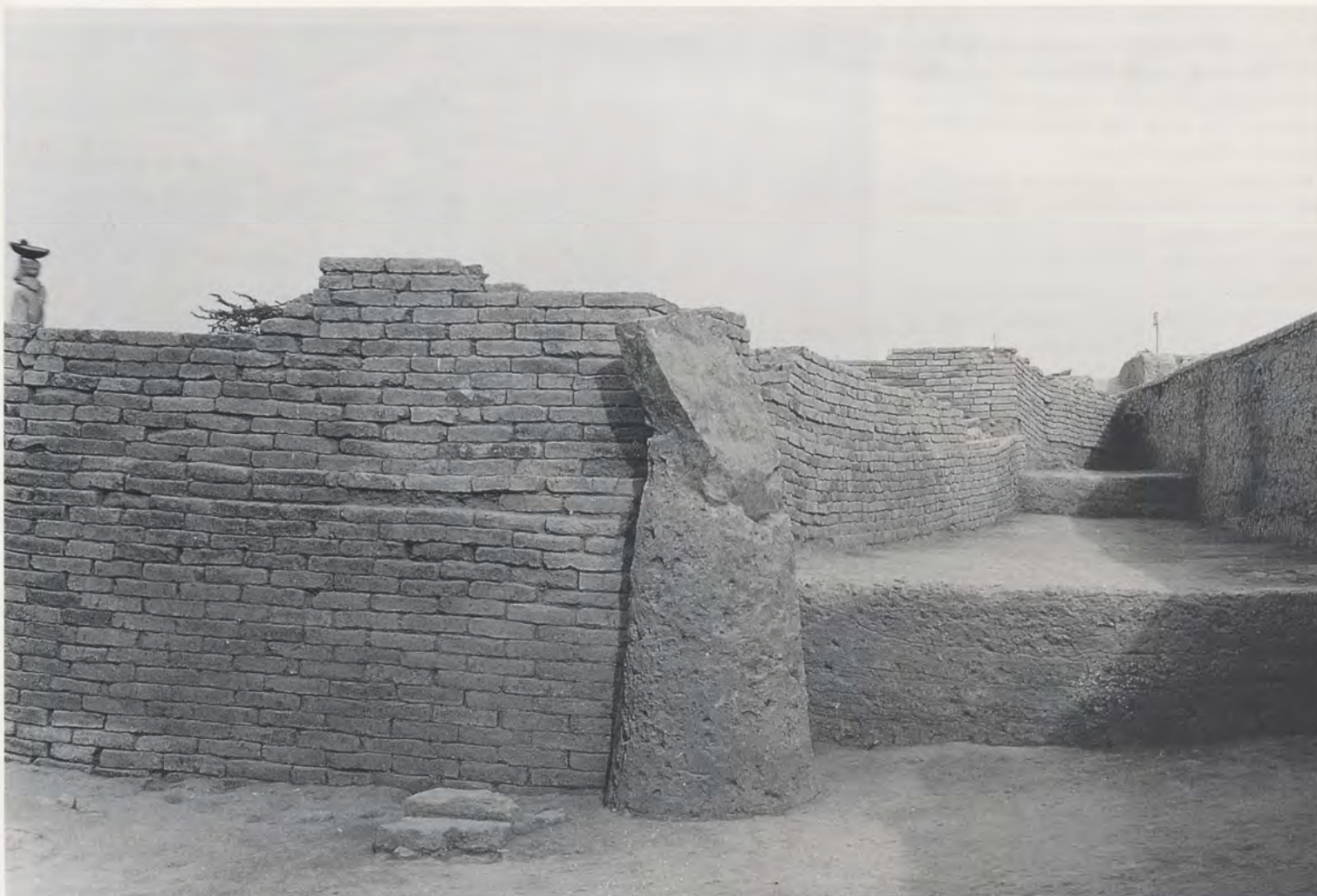
52 South-western corner of Block C with corner stone of Level 23 and superstructures of Levels 22–21
