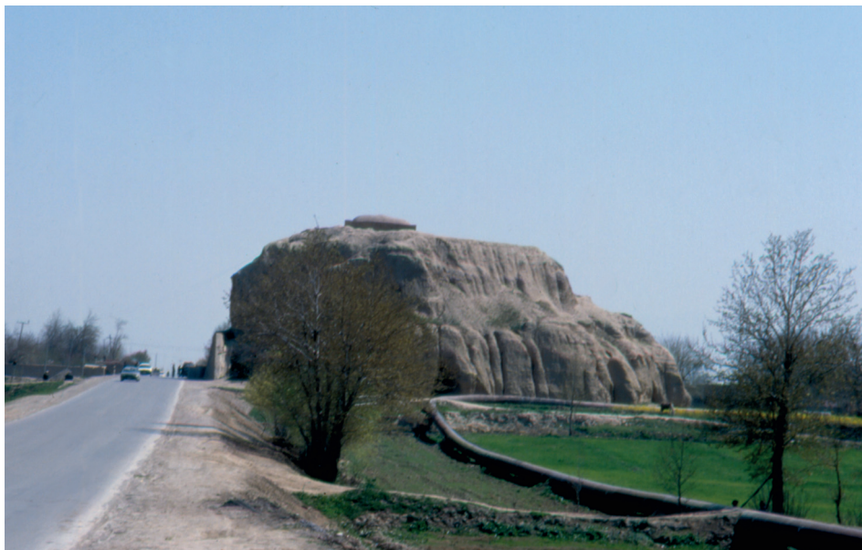
Fig. 1. A stūpa near Balkh (Bactra) damaged during the construction of the A-76 road (2003)
