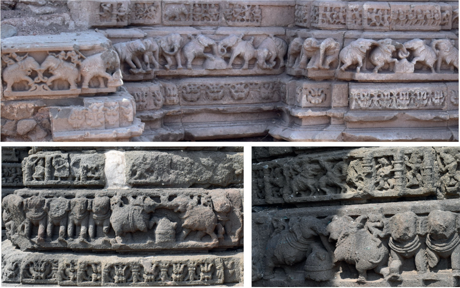
1. Base moulding, Shiva temple, Rajapura (upper), Base moulding Chaubar Dera II, Un (Lower).
