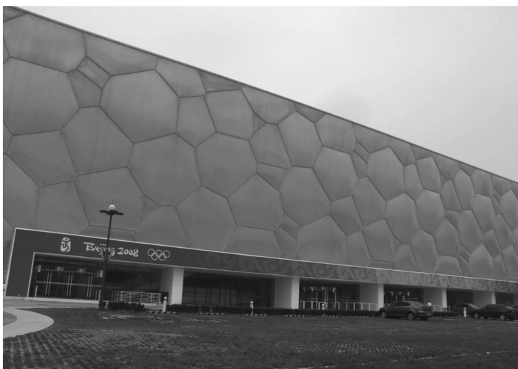
Fig. 5. PTW Architects (Australia), CSCEC International Design (China), ARUP, National Swimming Center – the Water Cube, Beijing 2003–2008 (photo J. Kucharzewska 2009)
