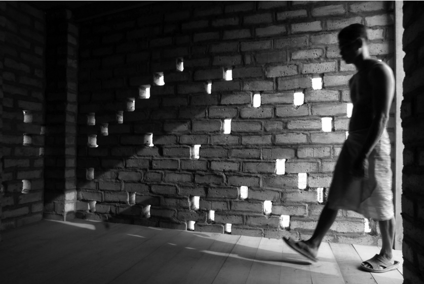
Fig. 5. Openings left between bricks providing natural ventilation. Image by courtesy of Architects Rudanko + Kankkunen
