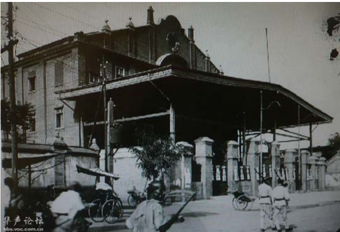
Ill. 11. Diyi wutai (The First Stage), opened 1914, was the first modern-style theatre in Beijing. With its construction made of bricks and timber it differed much from the traditional wooden teahouses. Source: [Diyi wutai], entry 15 July 2015
