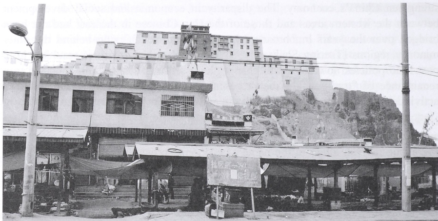
Fig. 2: Fort Shigatse, or “Concrete Castle”
