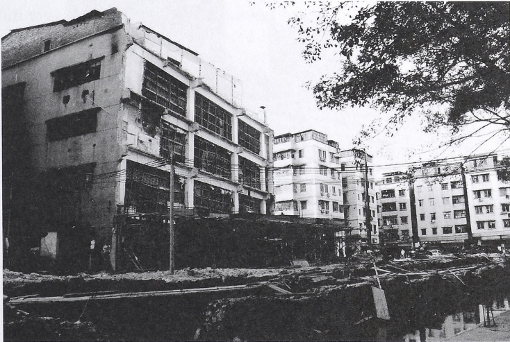
Figure 1: Demolition of a textile factory building in Zhongda textile district
