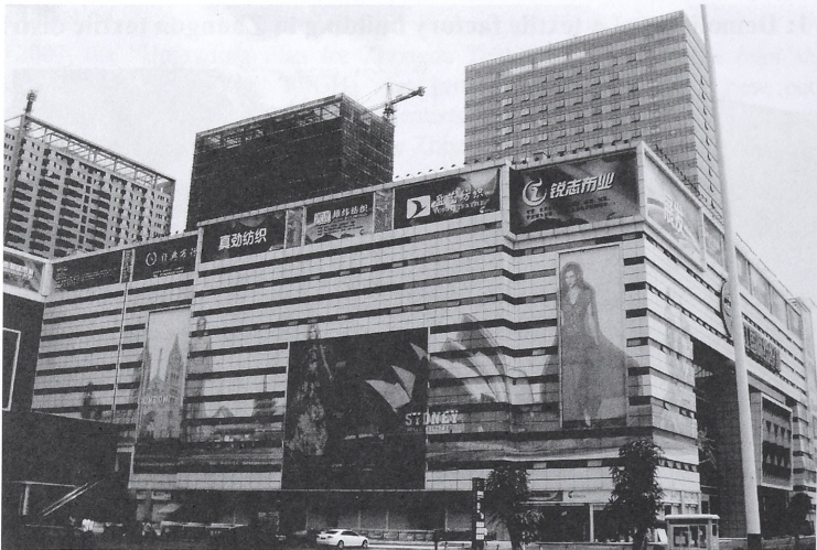
Figure 3: The Pearl River International Textile City main building
