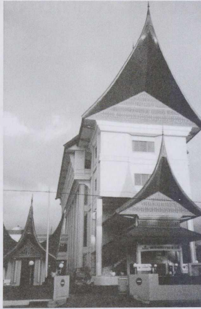
Figure 5: Bank Building, Padang, West Sumatra
