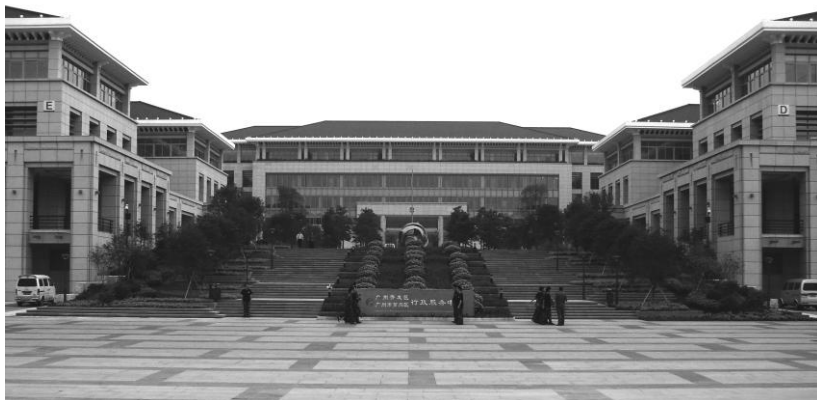
FIGURE 5: Joint headquarter of Luogang District and of GDD Administrative Committee
