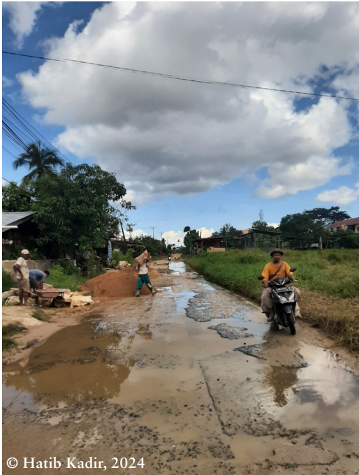
Figure 1: A road damaged by sand mining trucks
