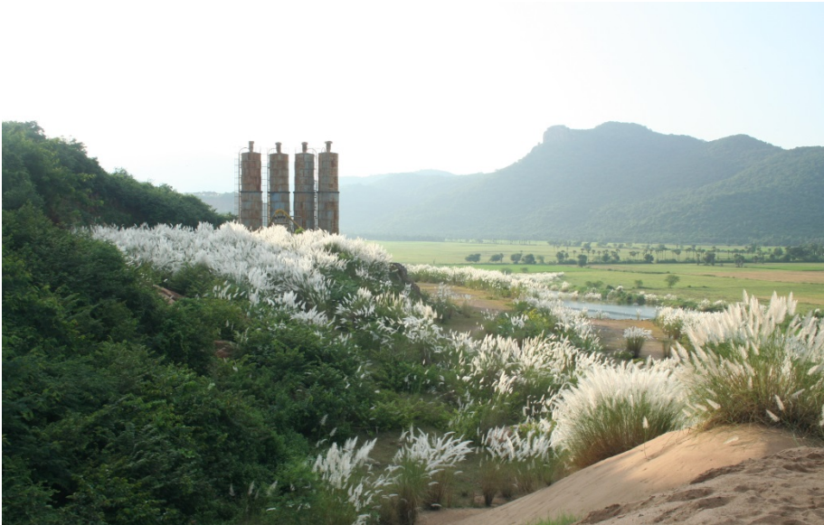
Photograph 1. Construction side of the dam wall and Godavari river (Photograph by Klara Feldes, September 2012).
